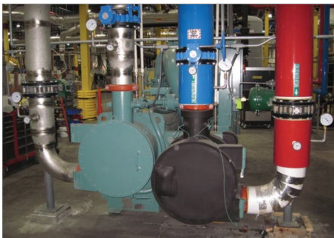
Examples of typical cooling system instrumentation: chiller gauges and line cooling gauges.
